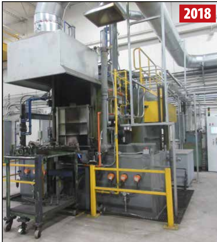
MIDLAND ROSS ALL-CASE 243624 LPG/METHANOL HEAT TREAT FURNACE
